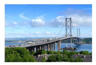
The Forth Road Bridge is one of the worlds' most significant long span suspension bridges. With a main span of 1006 metres between the two towers, it was the fourth longest in the world and the longest outside the United States when it opened in 1964. In total, the structure is over 2.5 km long. A staggering 39,000 tonnes of steel and 125,000 cubic metres of concrete was used in its construction.
